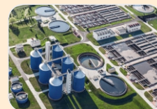
SEWAGE TREATMENT PLANT
