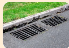
STORM WATER DRAINAGE
