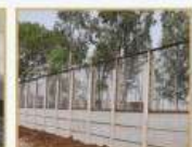
LAYOUT FENCING & DEMARCATION
